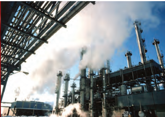
Instrumentation and Automated Pneumatic Controls
